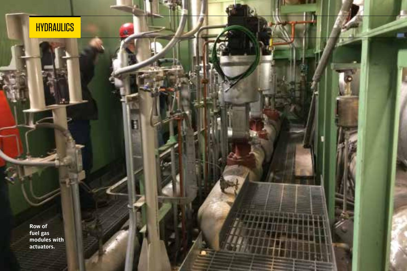
Row of fuel gas modules with actuators.
