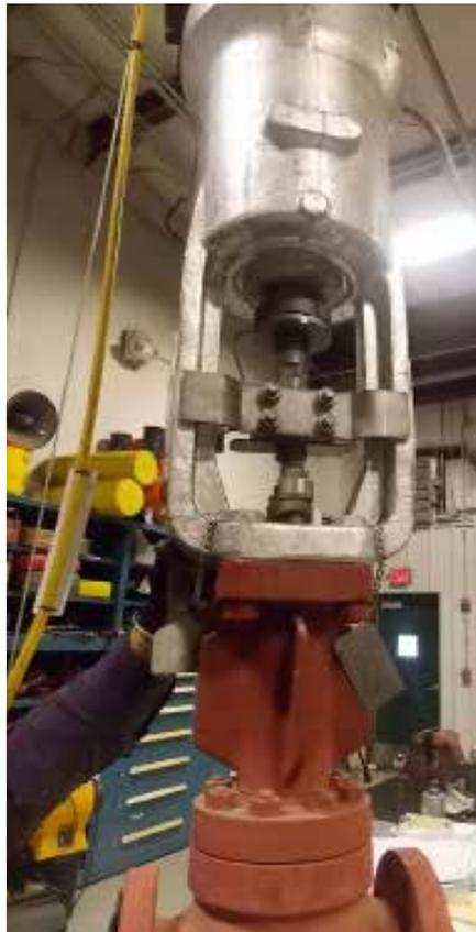
**Hydraulic actuator attached to a process valve.**
